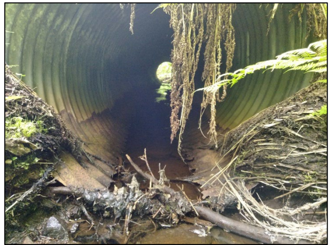
Figure 3.—Culvert just downstream of waypoint 471.
